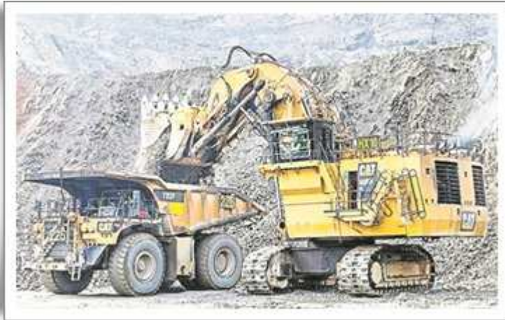
Mining operations in Ok Tedi Mine, Tabubil, Western. According to the MRA, the country's mining industry has done well over the years since the single operation on Bougainville in 1972. – Picture by Newcrest
