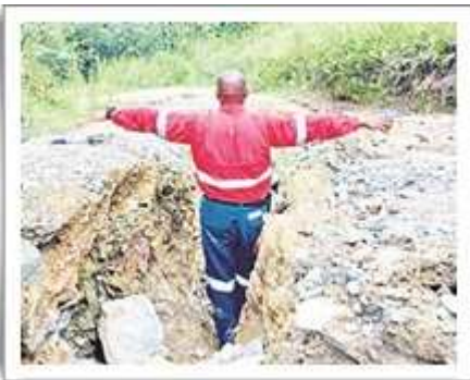
Part of the Wafi-Golpu road on Demakwa mountain. – Pictures supplied
