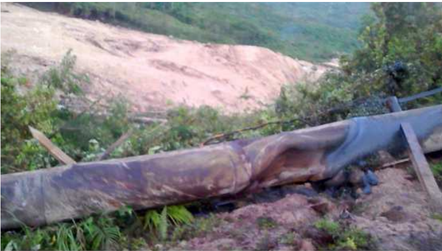
Landslide and damage to a road near the Ok Tedi mine. Jerome Kay/Handout via REUTERS
